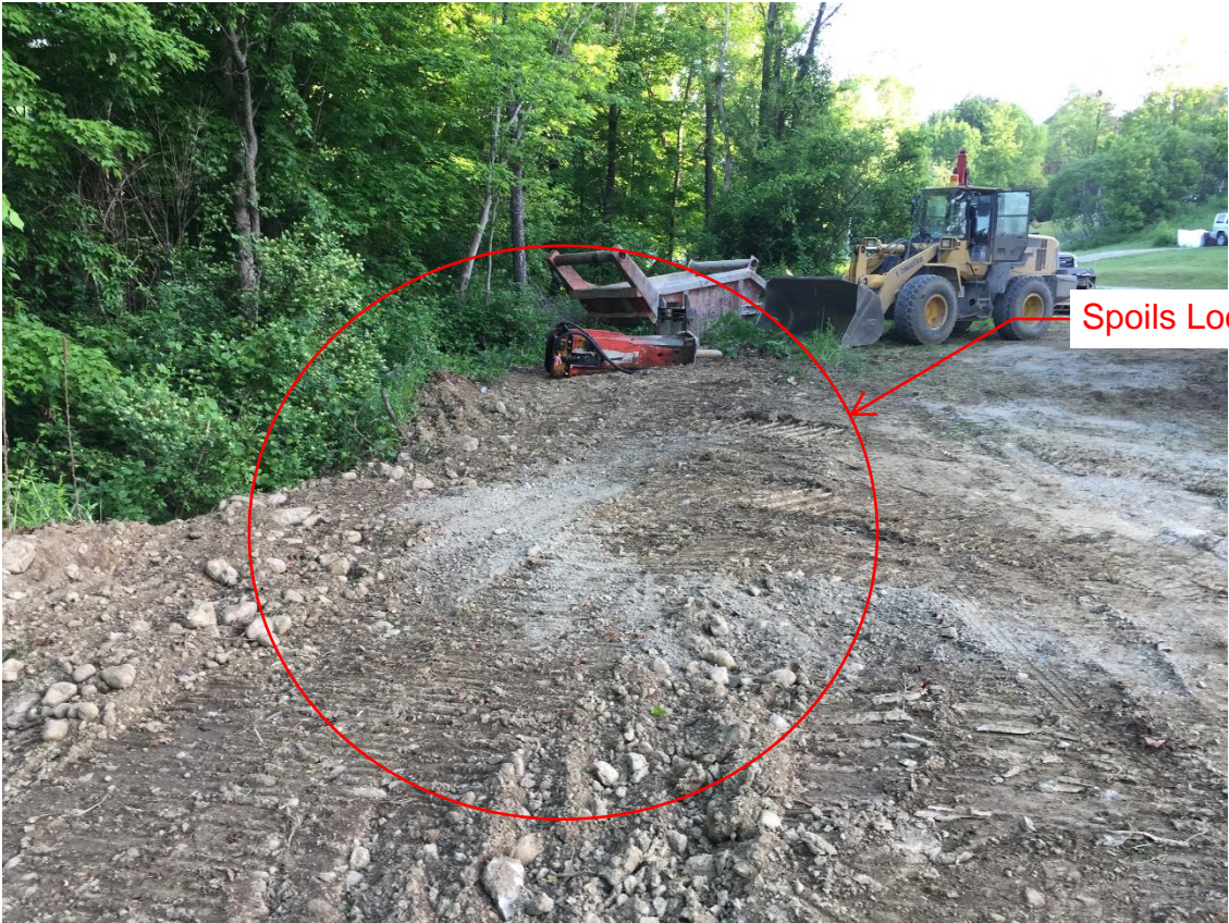
From west side of site, looking north
